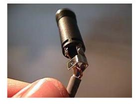
Clip off any excess wire that protrudes from the contact points (the white wire goes through the a hole, cut off the excess once it is soldered into place).
